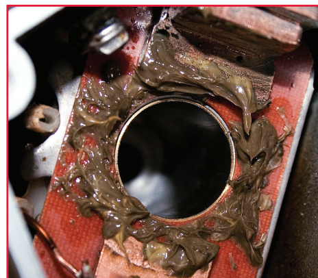
Grease applied to the solenoid contacts. This acts as an insulator and prevents current flow.
